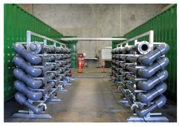
Two off skid mounted tube flocculators and containerised multimedia filtration plants
